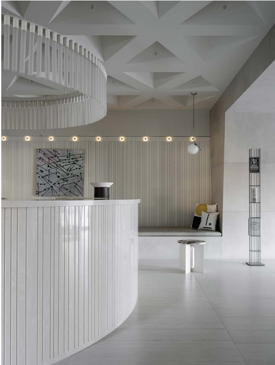
The triangular construction on the ceiling masks the ribs of the floor slabs. Painting by Clara Golitsina “Scattered.” Shelving, Mogg.
